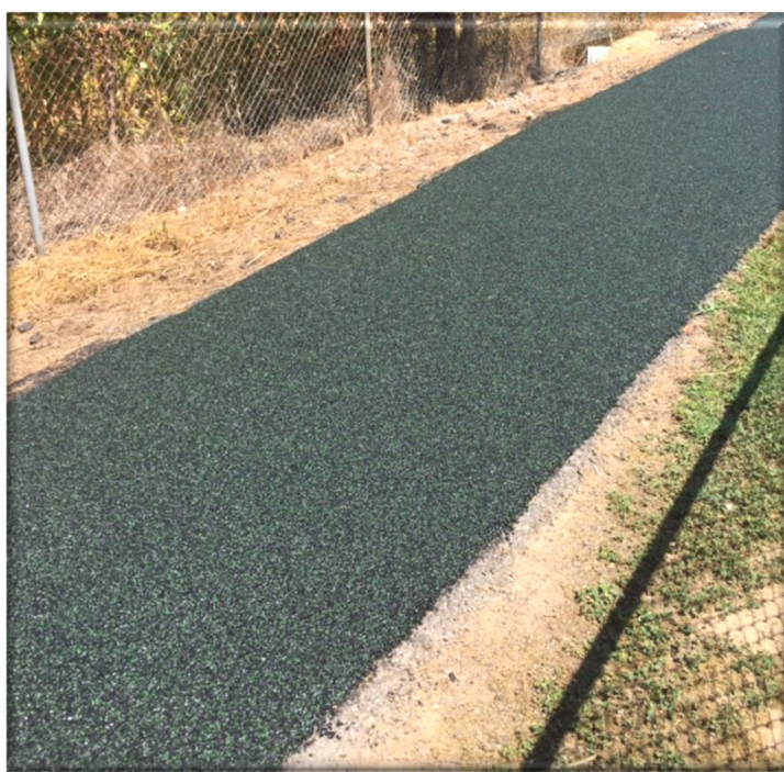
Photo 2: Crumb rubber pour-in-place walking trail, Green County Photo by Lisa Evans
